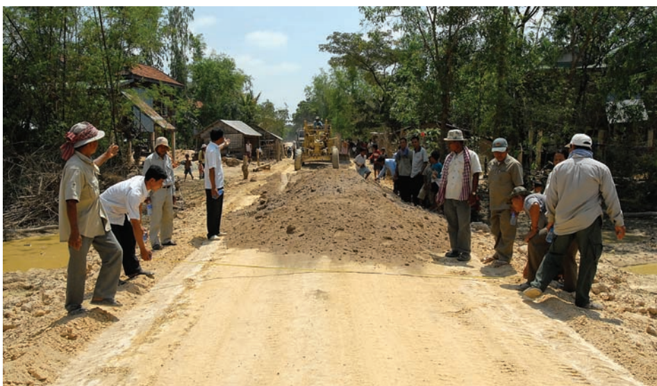
UNDP PHOTO Road construction in Cambodia.
